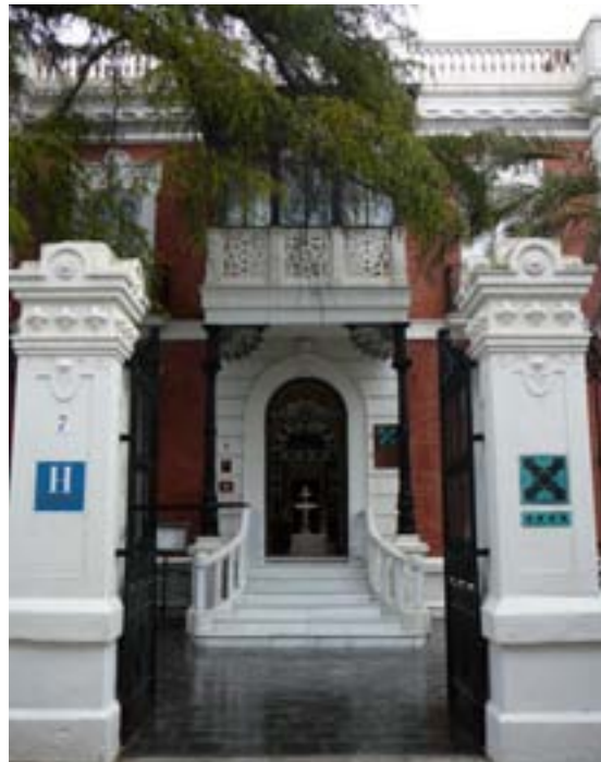
Photo 1 — Historic building converted into a four-star hotel (Spain)
