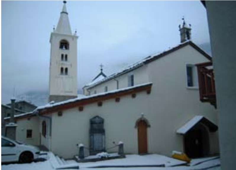
Photo 10 — Project involving the renovation of the exterior walls and roof of a church (France)
