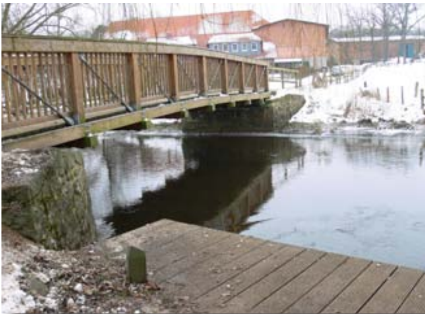
Photo 6 — Wooden bridge on a river to connect cycling and walking paths and a dock for canoes (Germany)
