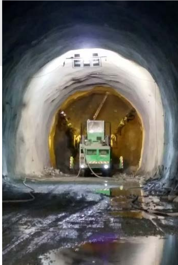
The explosives drilling truck
