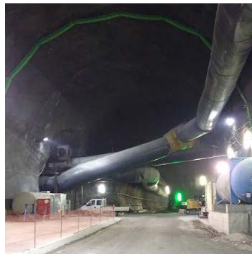
The cavern where the machinery is assembled
