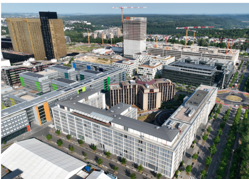
Figure 3 – Aerial view of the buildings in the European quarter
