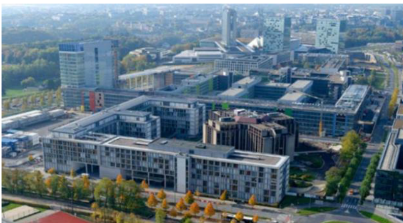
Figure 6 | Aerial view of the buildings in the European quarter
